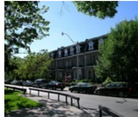
Residential facing onto Clarence Square.
