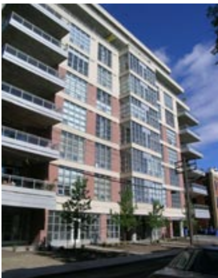
Most of the new development in the area has been condominiums.
