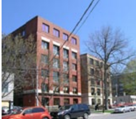
The historic buildings on Wellington support a diversity of uses.
