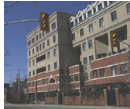
Recently constructed apartment condominiums on Richmond Street west of Spadina.
