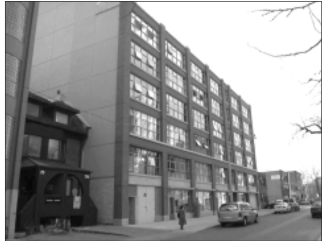
29 Camden Street, a new residential building based on an industrial facade treatment
