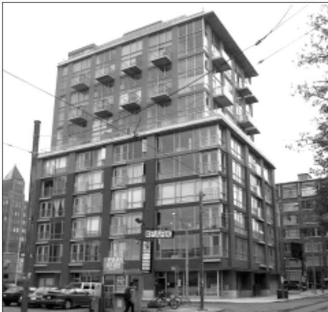
36 Charlotte Street, Charlotte Lofts, base building with predominantly glass floors above the setback
