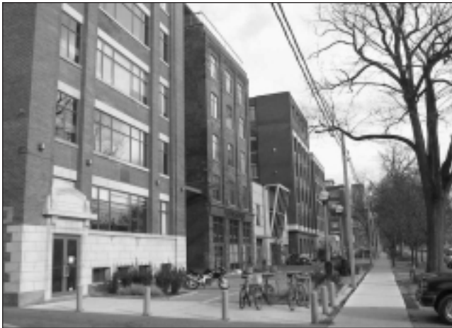
Renovated buildings and upgraded streetscape along Wellington Street West
